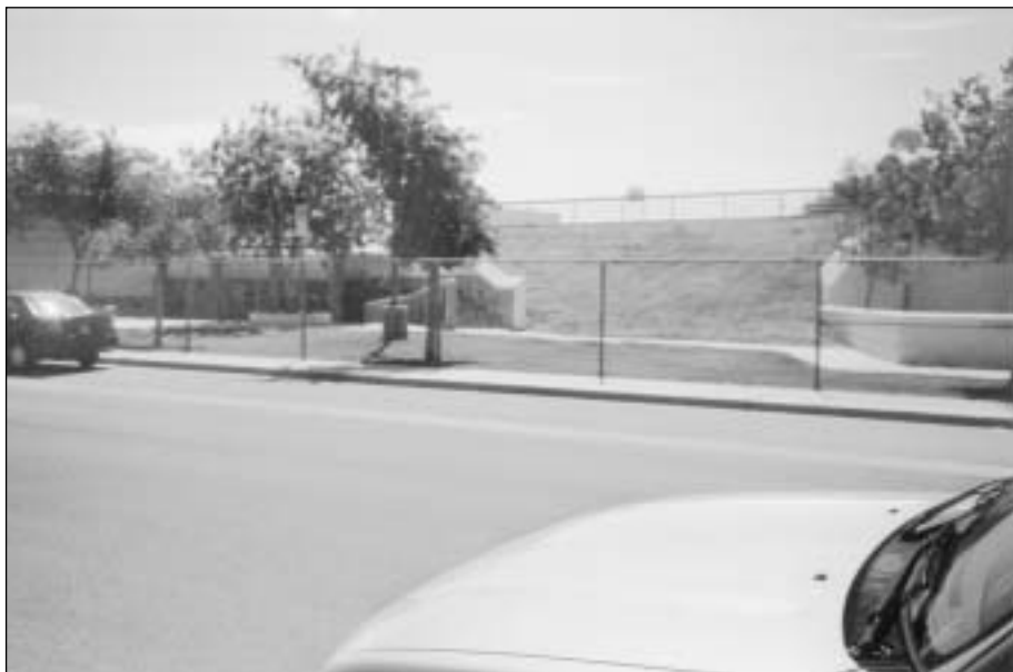
Luis helped to design the underground schools of Ann Ott and Herrera.
